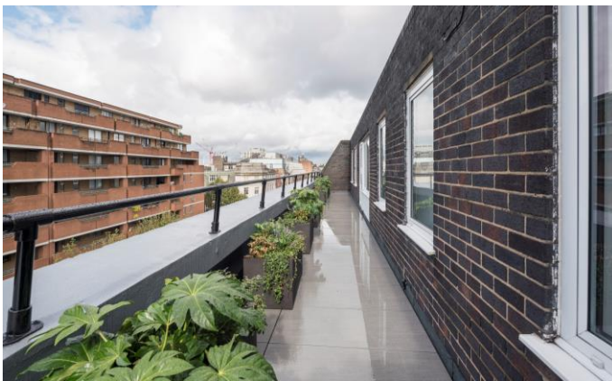
6th floor demised terrace
